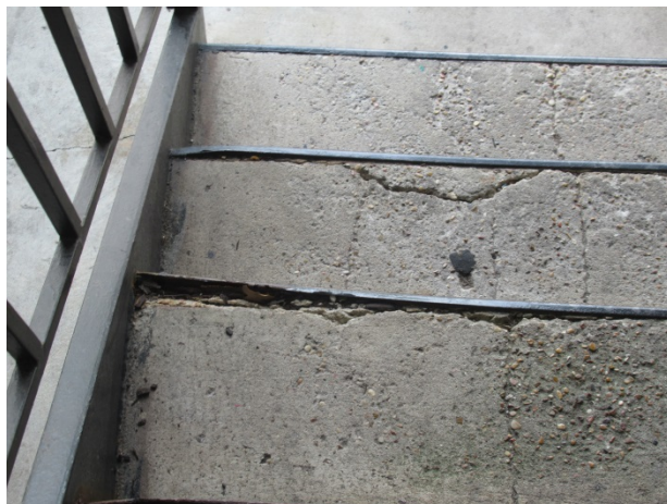
Concrete cracks and damaged frame
