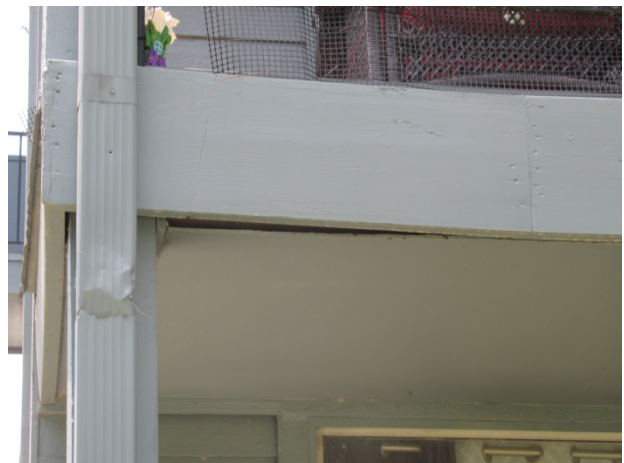
Damaged soffit
