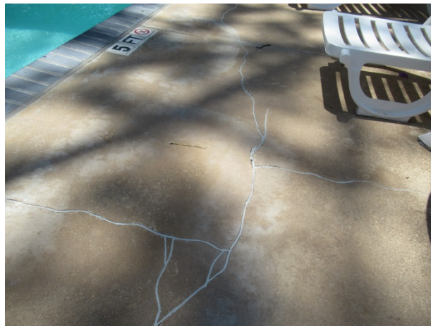
Previous crack repairs
