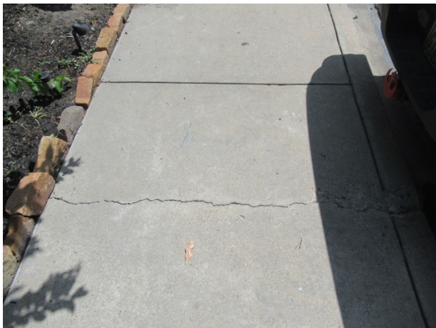
Concrete cracks
