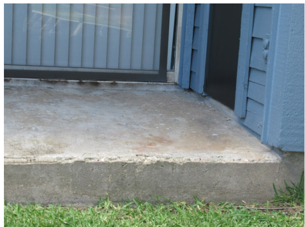
Spalled concrete
