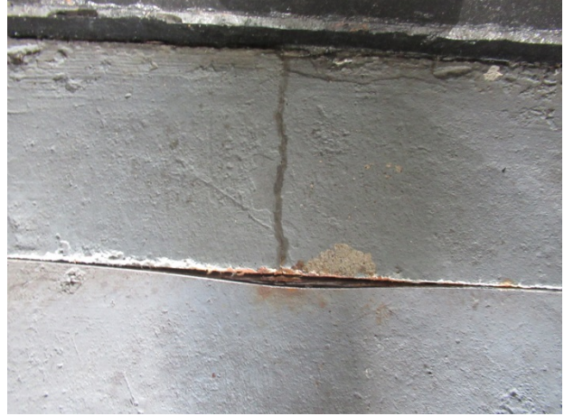
Rust and damage at frame
