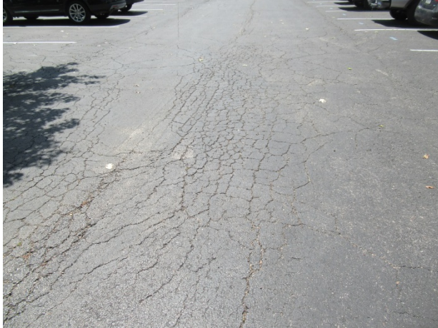
Alligator cracks
