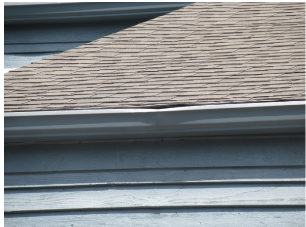
Dented gutter
