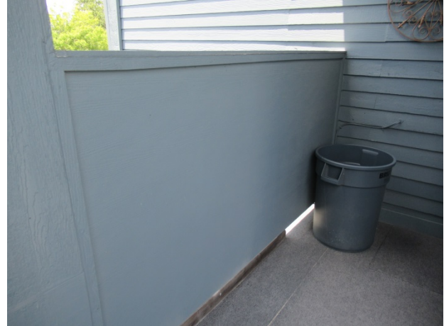
Recently installed fiber cement railing at breezeway
