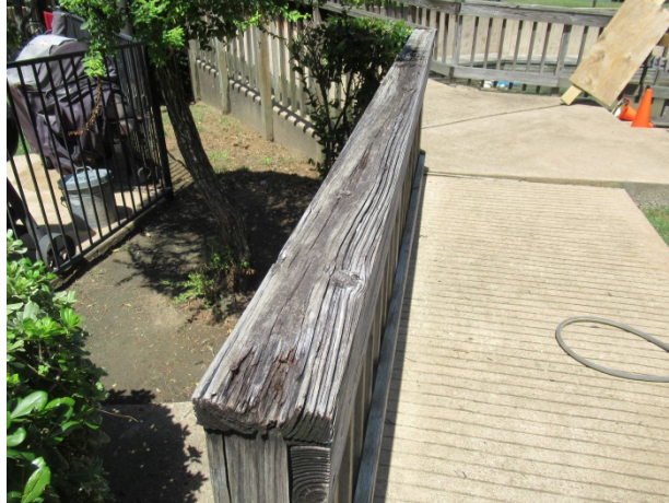
Weathering of wood at railing
