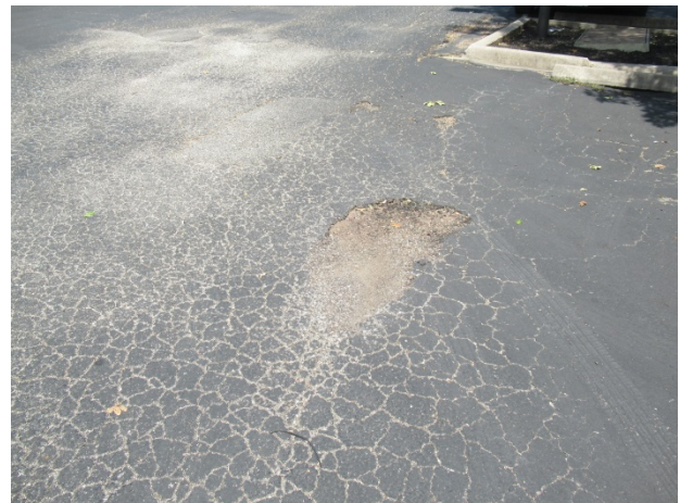
Pavement deterioration and alligator cracks
