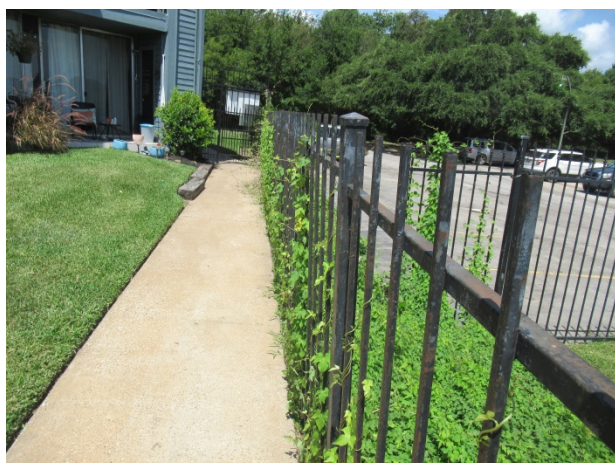
Finish deterioration and rust
