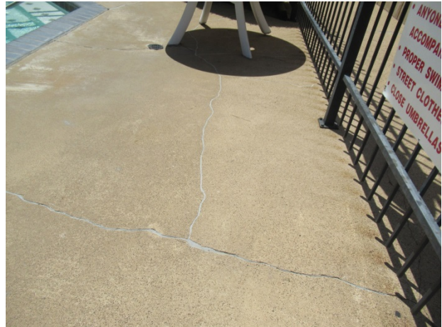
Previous crack repairs
