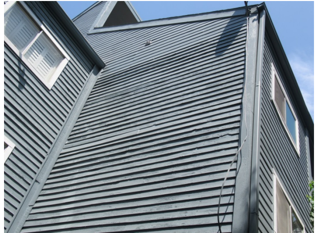
Weathered and deflected siding
