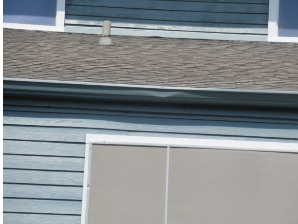
Dented gutter
