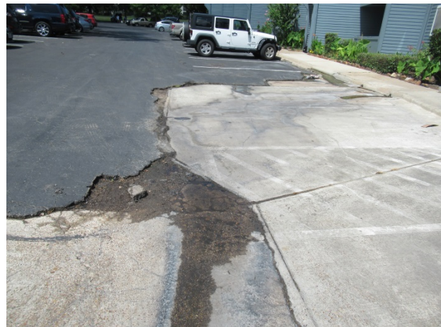
Section patched with concrete
