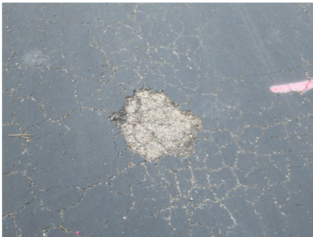
Pavement deterioration and alligator cracks
