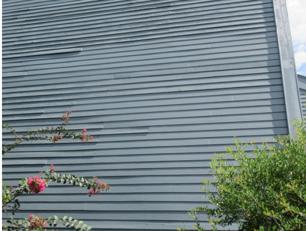
Loose and weathered wood siding – Note sections replaced with fiber cement siding
