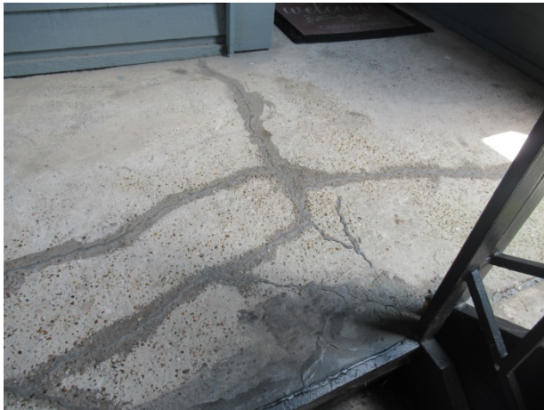
Previous crack repairs
