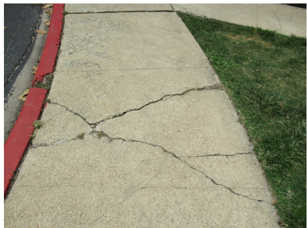
Concrete cracks
