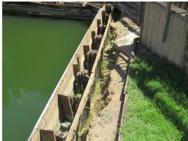
Section of bulkhead being replaced in 2020
