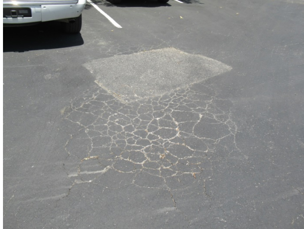
Alligator cracks around previously patched section
