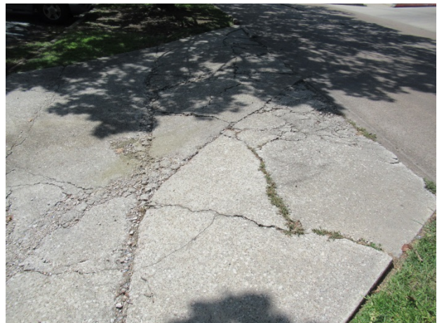
Concrete cracks and damaged by the trash corral
