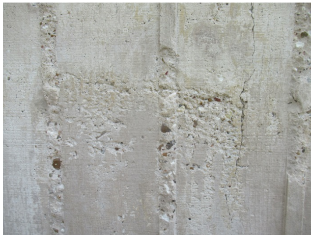
Spalled concrete
