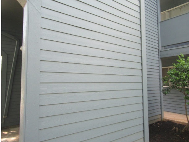
Recently installed fiber cement siding
