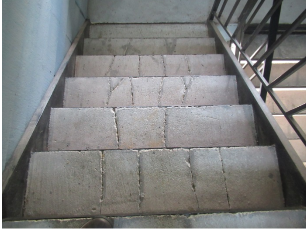
Concrete cracks
