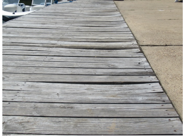
Loose and deflected deck boards
