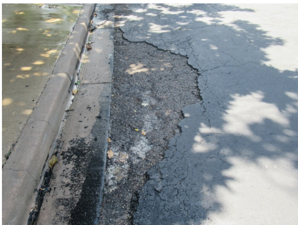
Deterioration of the overlaid top course
