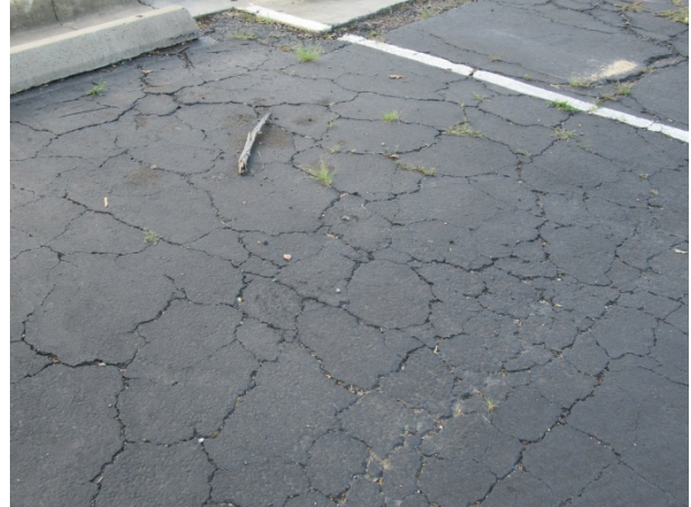
Alligator cracks
