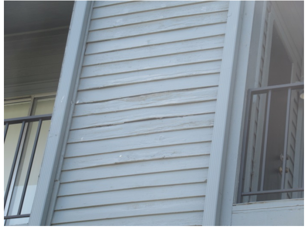
Weathered and damaged siding
