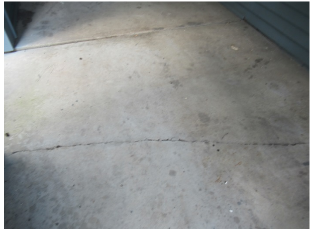
Concrete cracks
