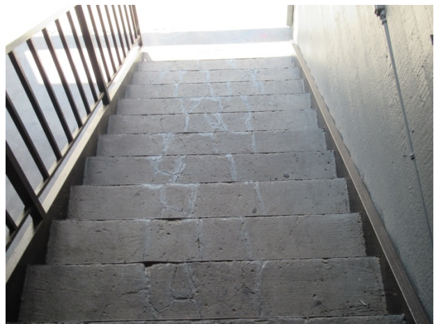
Previous crack repairs at concrete treads
